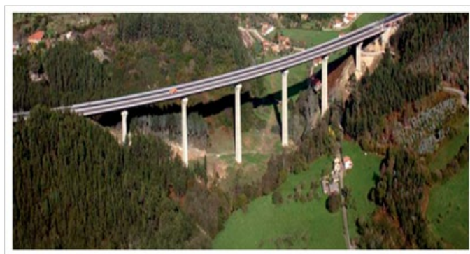
Concrete quality control in civil engineering
