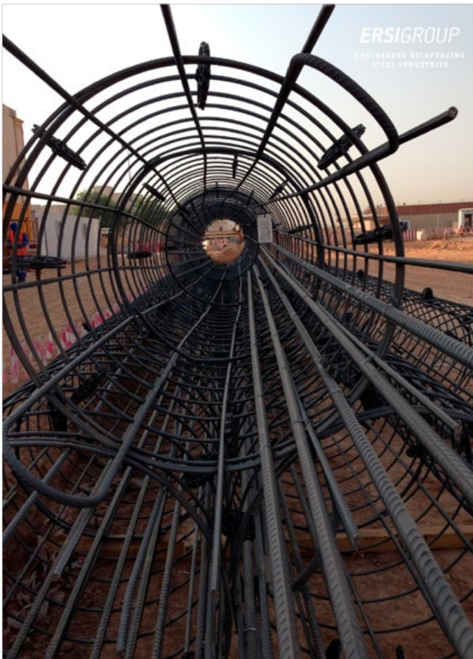
Reinforcing steel required for the construction of the corresponding asymmetric pile.
